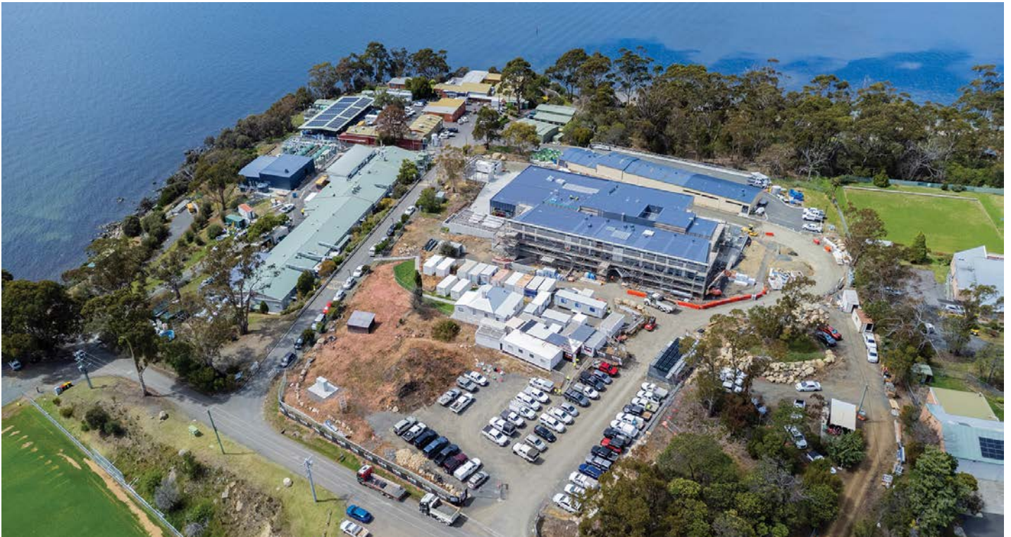
Bird's eye view of the construction at IMAS Tarooma. Credit: Peter Allen
